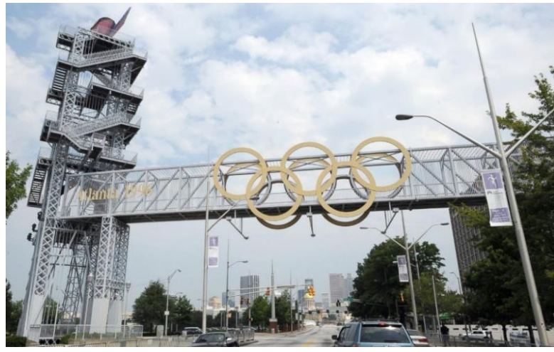
Figure 2.5 1996 Olympic Games Bridge on Capitol Avenue (Lesser, n.d.)
